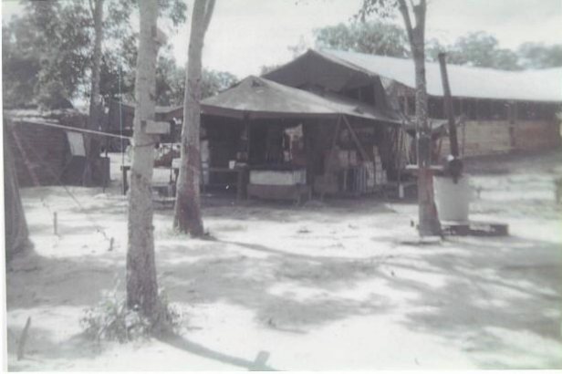
Figure 1 - A Company's Mess Hall – Cu Chi 1966.
